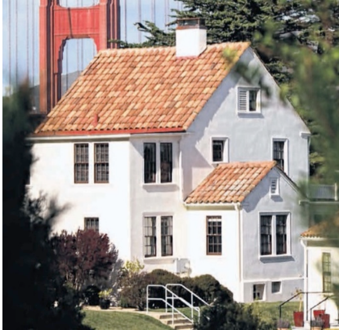
Cool roofs & walls
